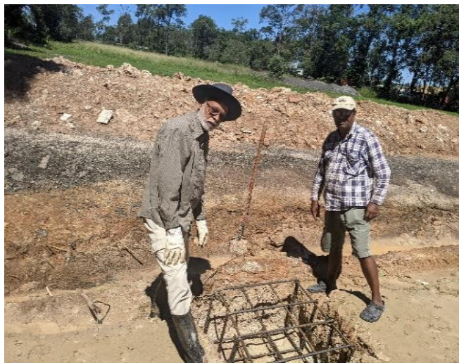
Gone in place
