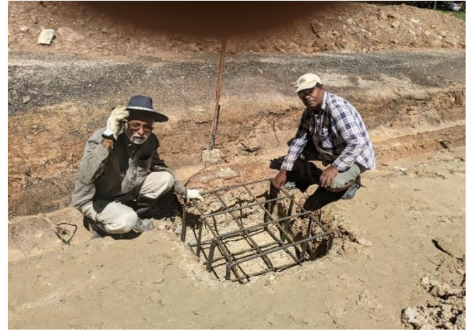
Steel Post Footing Going ..... Going .....
