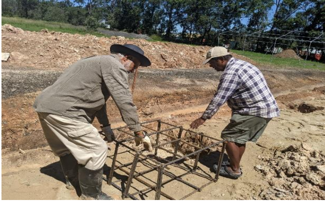
Steel Post Footing Going ..... Going .....
