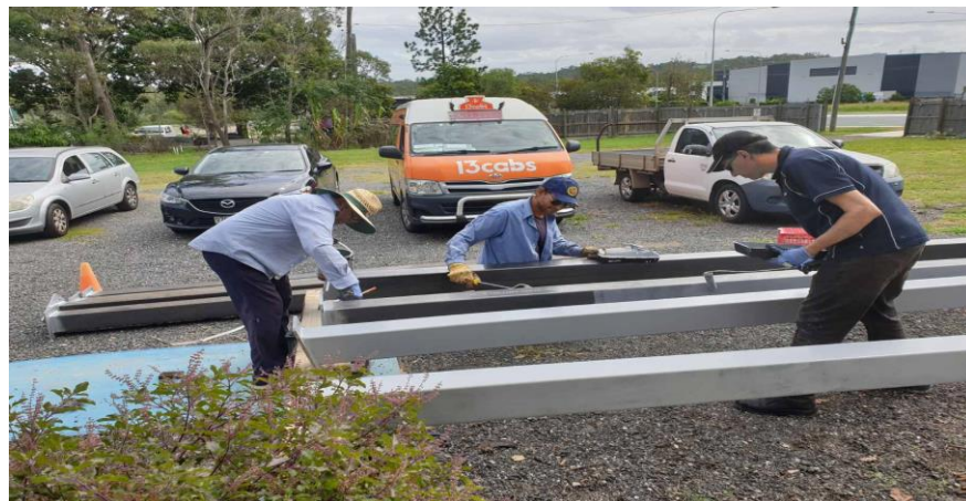
Steel posts being cleaned and rust proofing done.....
