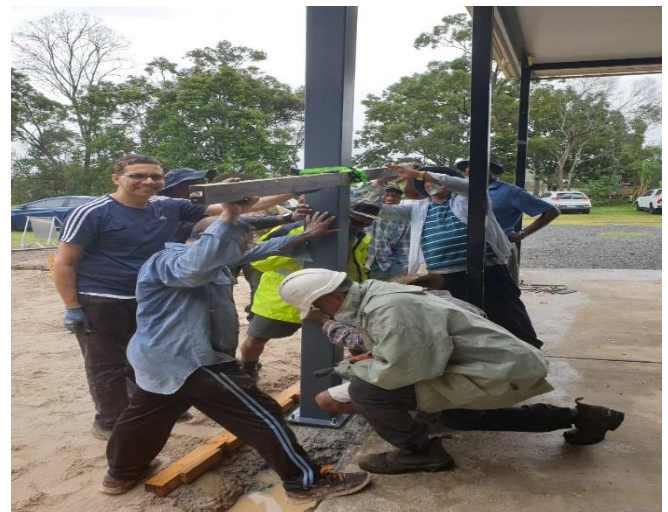
First Steel post lined and in place
